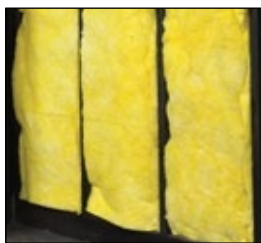
R-11 insulation in walls, ceiling, and sump walls
