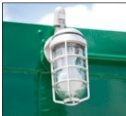
Vapor-resistant exterior light with photocell
